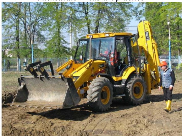
Buldoexcavator JCB 3CX – lucrări practice
