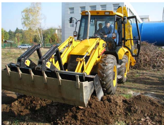
Buldoexcavator JCB 3CX – lucrări practice
