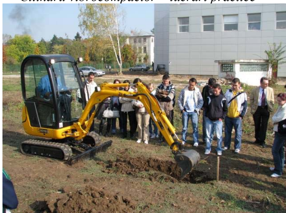
Miniexcavator – lucrări practice
