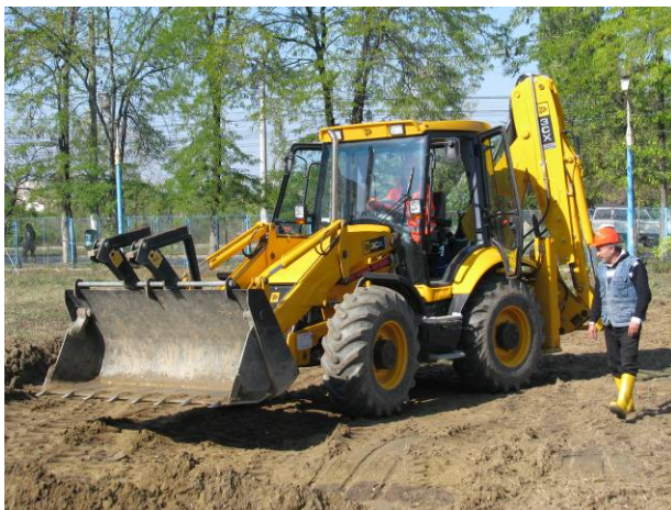
Buldoexcavator JCB 3CX – lucrări practice
