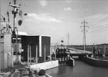
Complexe station de pompage
